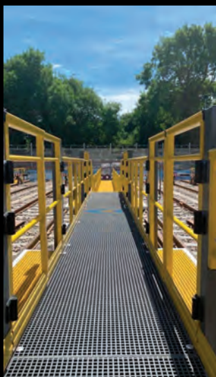
Driver Access Platforms
