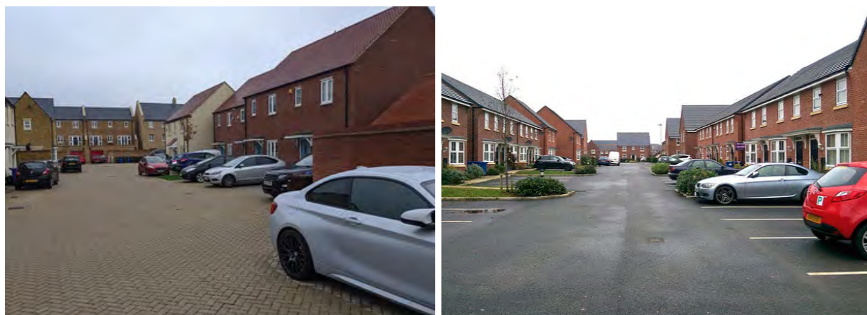
The car is still king in these new build suburban developments in Chapelford, Warrington and Bicester, Oxfordshire. Images: Transport for New Homes
