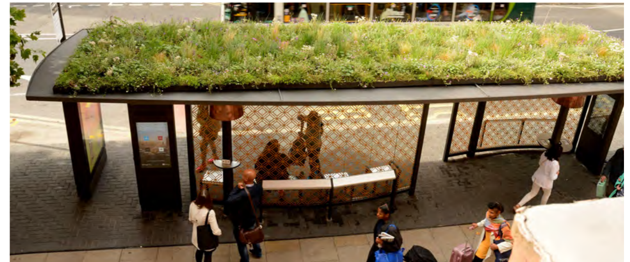
An example of a bus shelter with green roof in Manchester City Centre. Image: Transport for Greater Manchester
