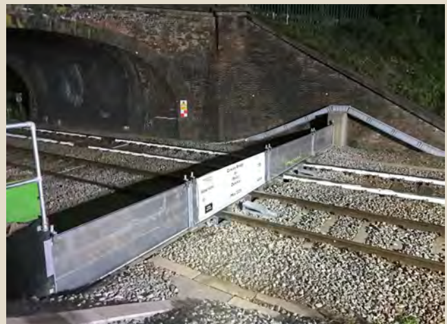
Network Rail’s flood defence barrier to stop flooding north of Exeter was brought into use in May 2020. It can be quickly assembled across the line when poor weather is forecast. NETWORK RAIL.
