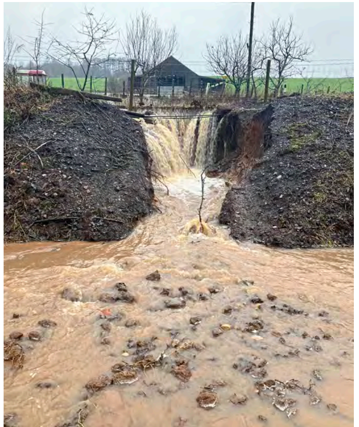
Flooding will become a particular challenge. In December 2023, the Glasgow & South Western route from Carlisle was severed at Thornhill, when large volumes of water overwhelmed a culvert, leaving track suspended over the gap. More than 100 tonnes of debris fell across the track between Dumfries and Sanquahar. NETWORK RAIL.
