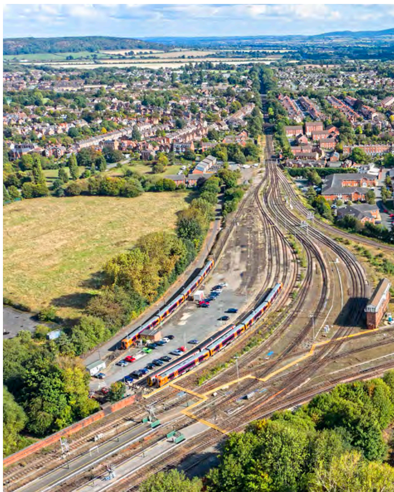
An aerial view of Shrewsbury Bridge Junction, from where routes to Wolverhampton, Chester and Crewe, mid-Wales and the Welsh Marches all diverge. Sufficient funding is expected to be earmarked to protect the resilience of key junctions like this. TOM MCATEE.
